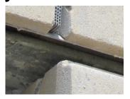
Weep holes located on top of mortar above flashing does not work and will create a wall issue due to water storage!
